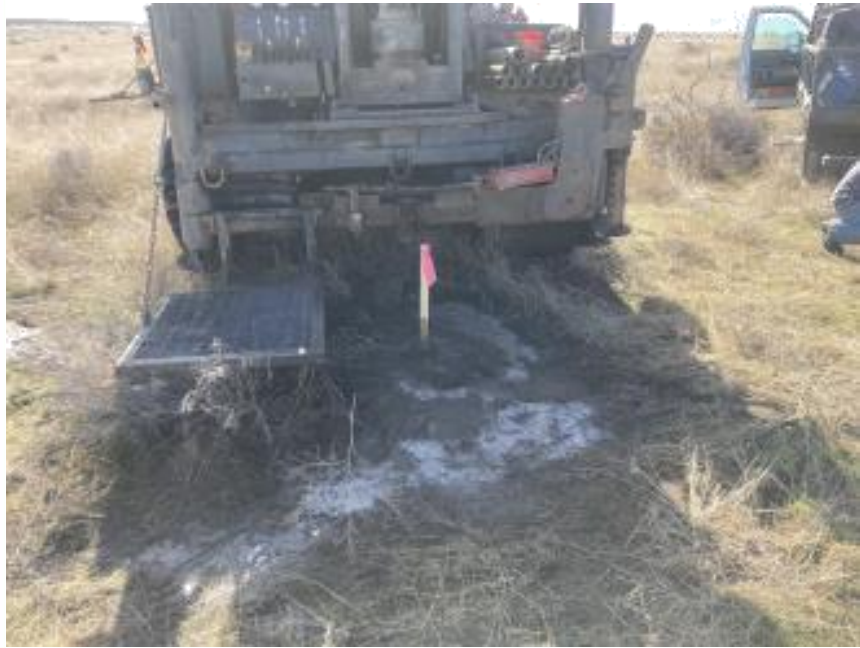
Photo 2 - Example of bentonite-backfilled borehole
