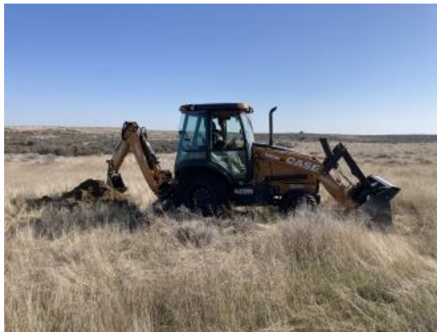
Photo 4 - Excavator used for digging test pits
