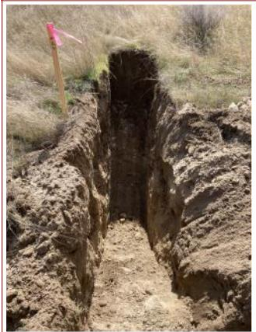
Photo 5 - Test pit location
