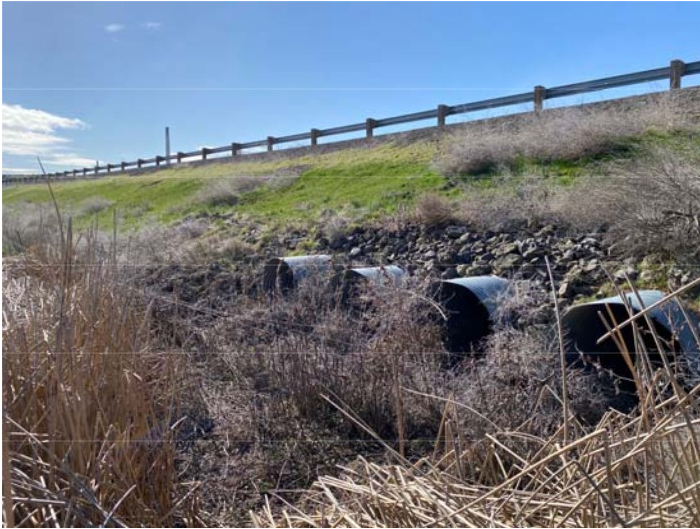
Photo M. View of 4 culverts under Tower Road draining into Interim Water 1 at March 31, 2022 site visit. No flow or surface water was present.
