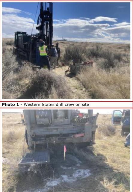
Photo 2 - Example of bentonite-backfilled borehole
