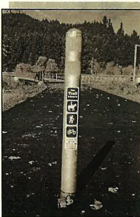
Figure 68. Bollard placed to prevent motorized access.
