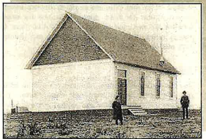
Figure 82. Turn of the century photograph of Irrigon (courtesy of Don Eppenbach).
