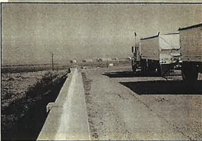
Figure 48. East Columbia Avenue railroad overpass
